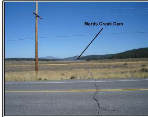
Photo 8: Looking north from Highway 267 to Martis Creek Lake and dam
